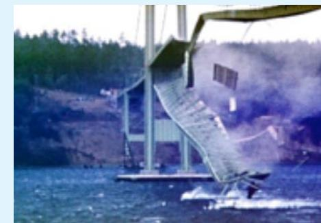
**Figure 5.2:** The effect of wind-induced resonance on an ill-designed structure.
