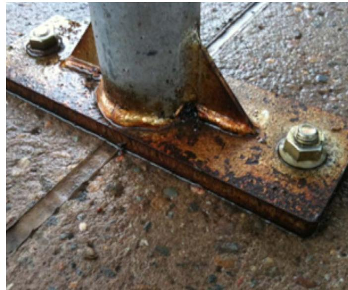
**Figure 6.7:** The effects of galvanic corrosion as a result of incompatible metals in contact.
