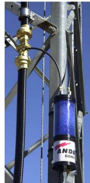
Dehydrator with waveguide
