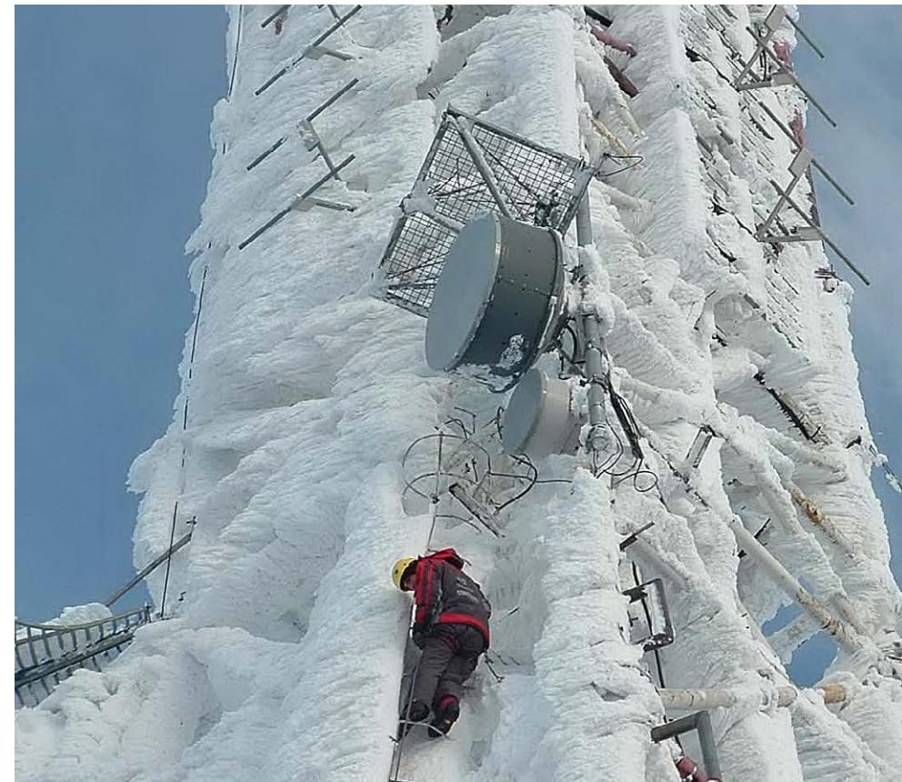
**Figure 5.4:** Ice buildup can mean falling ice and damaged antennas.
